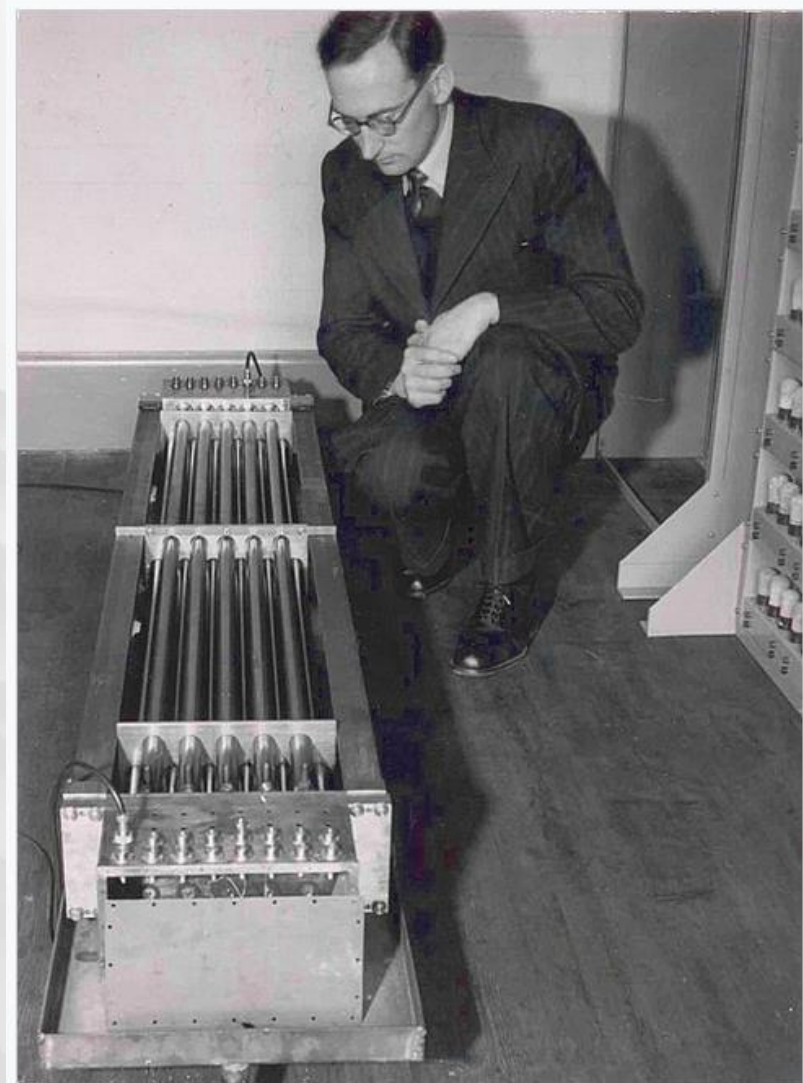
Maurice Wilkes inspecting the mercury delay line of the EDSAC in construction
